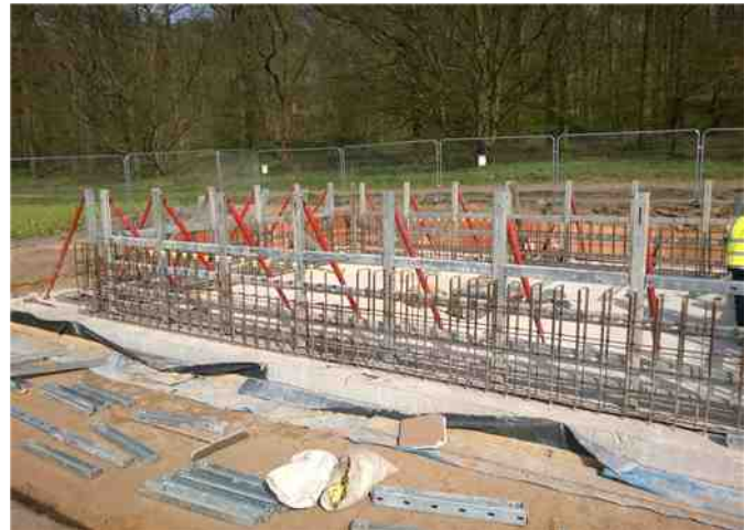
1.9m / 2.4m & 3.2m in use on retaining wing wall
