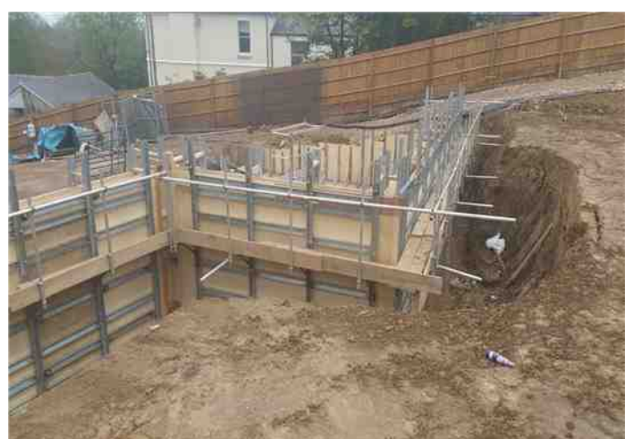
1.9m / 2.4m & 3.2m in use on retaining wing wall
