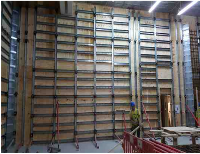
6.4m high hand fit steel system for Google, London
