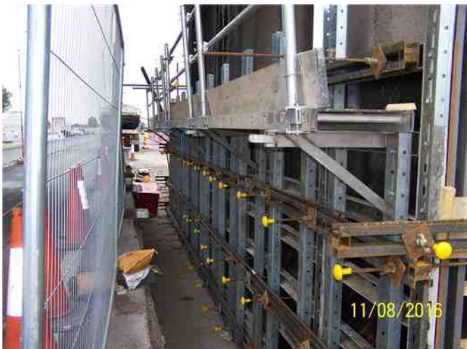
Aluminium system in use on M6 Smart Motorway upgrade
