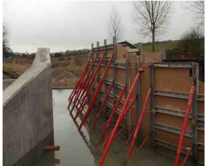
Battered wing walls for Amco flood alleviation scheme
